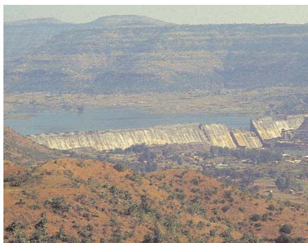
▲ Water and power sectors need to focus much more on decentralised sources, rather than on destructive mega-projects
