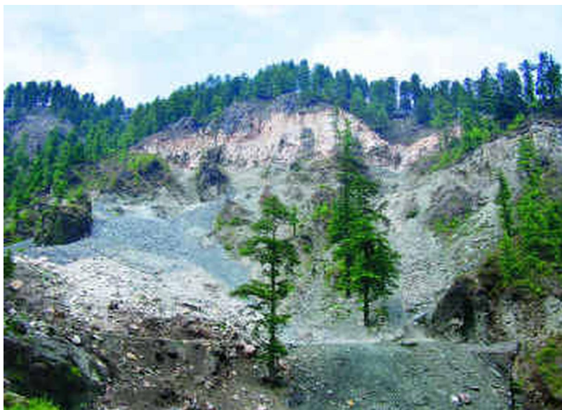
Destruction wrought by the Parvati hydroelectric project in Himachal Pradesh.-ASHISH KOTHARI
