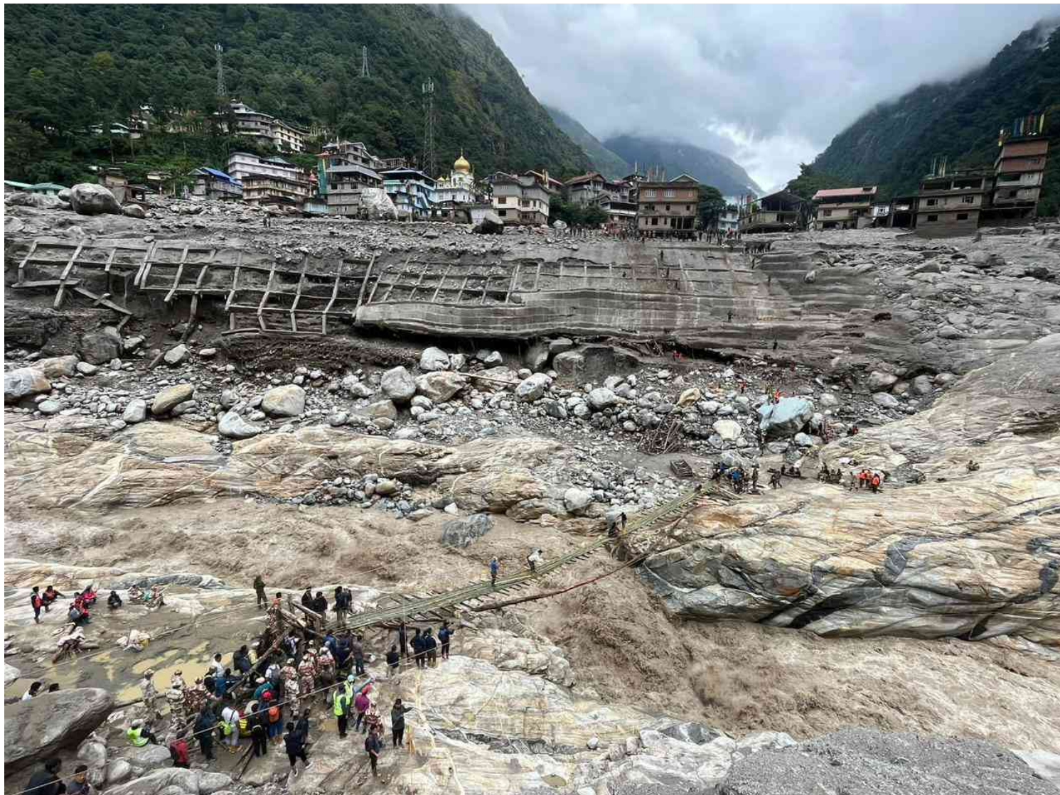
A temporary bamboo bridge being set up at Chungthang, where the Teesta III dam was swept away. Credit: Government of Sikkim/Facebook.
